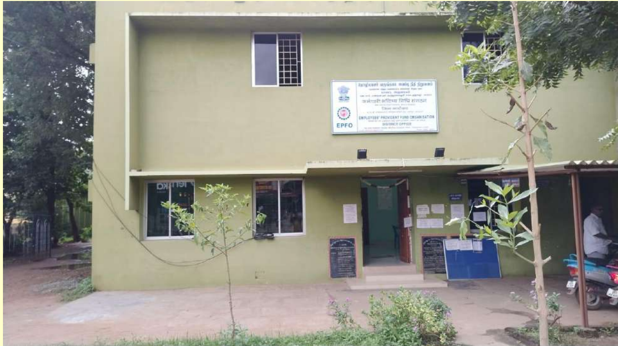
District Office Thanjavur
